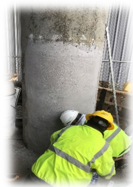
Vertical Column Repair
