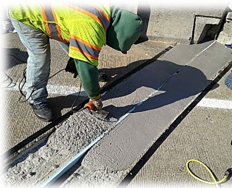
Expansion Joint Header Installation
