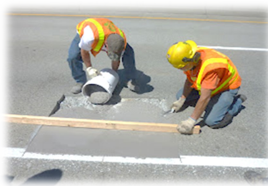
Bridge Deck Spall Repair
