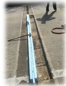
Use Foam Board to Establish Expansion Joints
