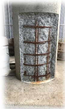
Vertical Column Site Preparation
