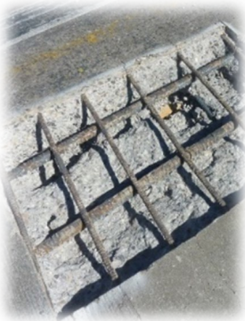
Deck Spall Ideal Site Preparation
